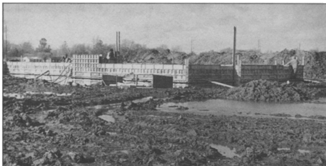
Foundation work on December 3, 1986
